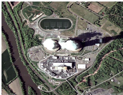
◀ The Limerick Generating Station in Pennsylvania uses two natural draft cooling towers (center) to remove heat during normal operation and a pond with water sprays (oval at upper left) as the UHS during accidents for the two reactors below the cooling towers.
