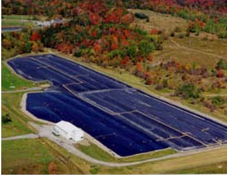
Figure 13. Aerial View of SDA 111
