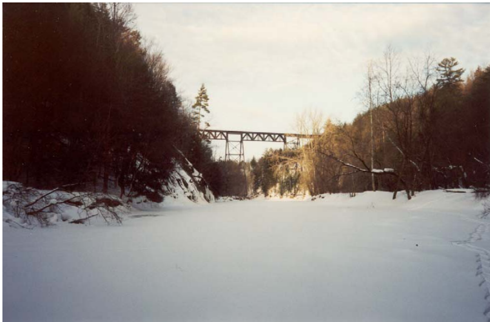
Figure 10. The bridge over Cattaraugus Creek, used to transport materials into and out of West Valley until 1998, was originally built in 1898. 59
