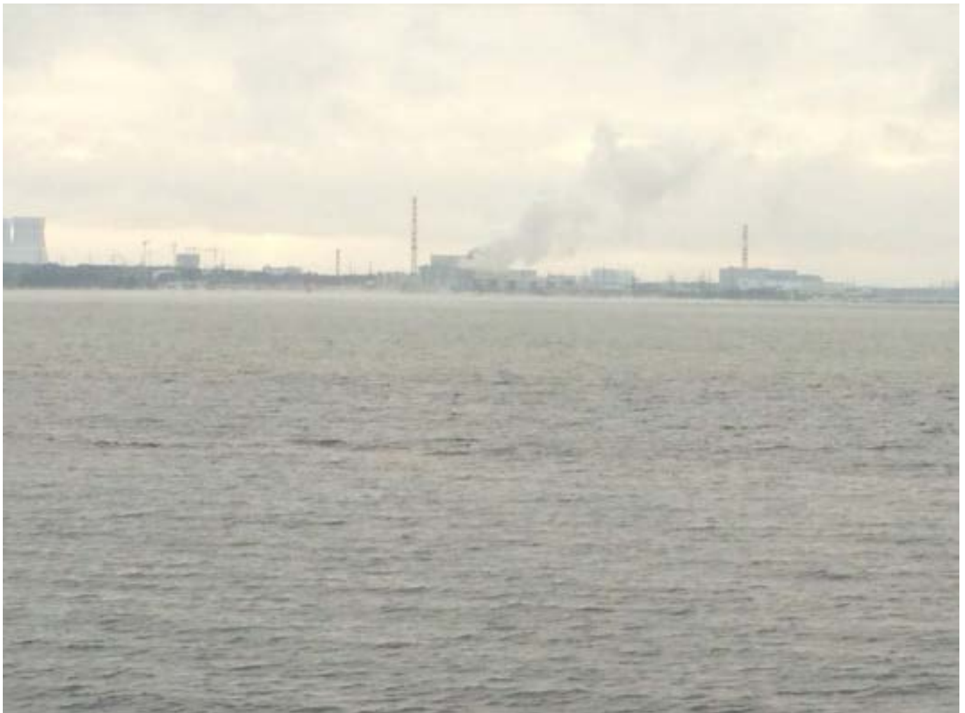
Photo of the radioactive steam blowing in the direction of Vyborg.
