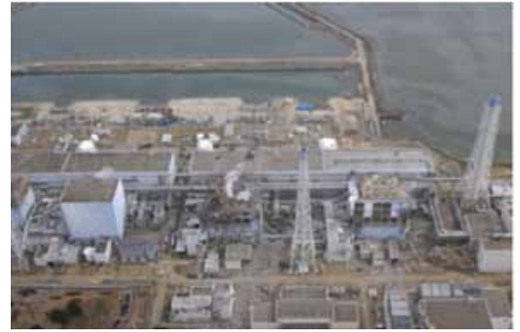
▲ Views of the reactor buildings following the explosions
