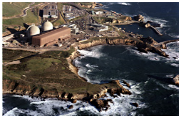
The “once-through” cooling system at California’s Diablo Canyon nuclear complex, as at many other reactors, discharges water (see plume in photo) at a much higher temperature than brought in, killing large amounts of fish and devastating other marine life.
