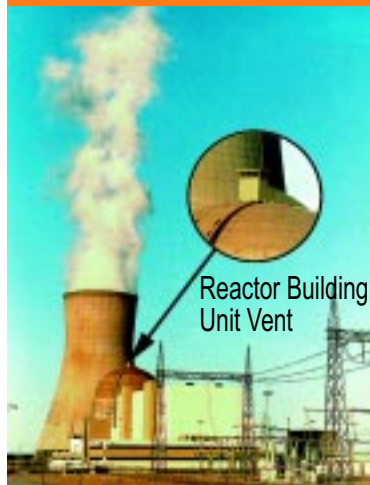
A Reactor Building vent at a typical 1000-megawatt pressurized-water reactor.
