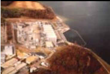
The 845-megawatt Calvert Cliffs reactors are the first in the U. S. to be relicensed for an additional 20 years.
