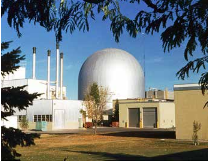
The EBR-II reactor in Idaho – the prototype ‘integral fast reactor’.
