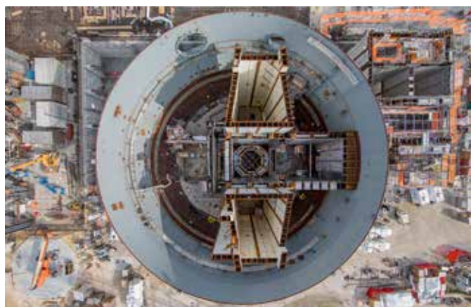
Vogtle unit #4 under construction in Georgia.
