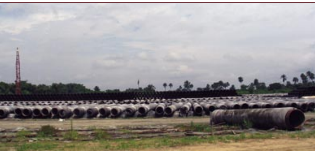
Pipes for the Nigeria-Ghana gas pipeline.
