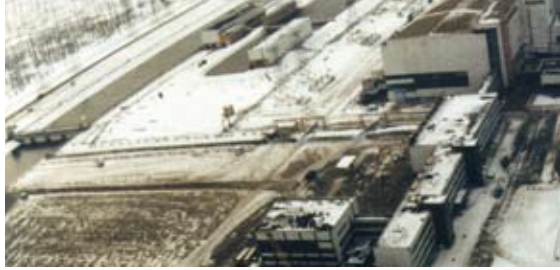
In Chernobyl two reactors are still in operation. Source: Natalia Manzurova
