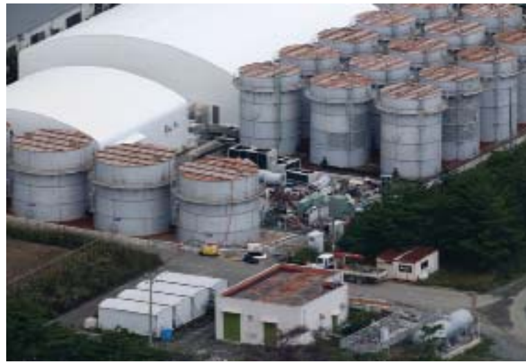
Water storage tanks at Fukushima.
